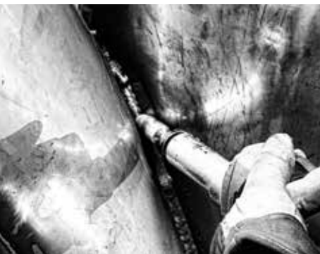
Cleaning a weld joint with a controlled flare end brush.
